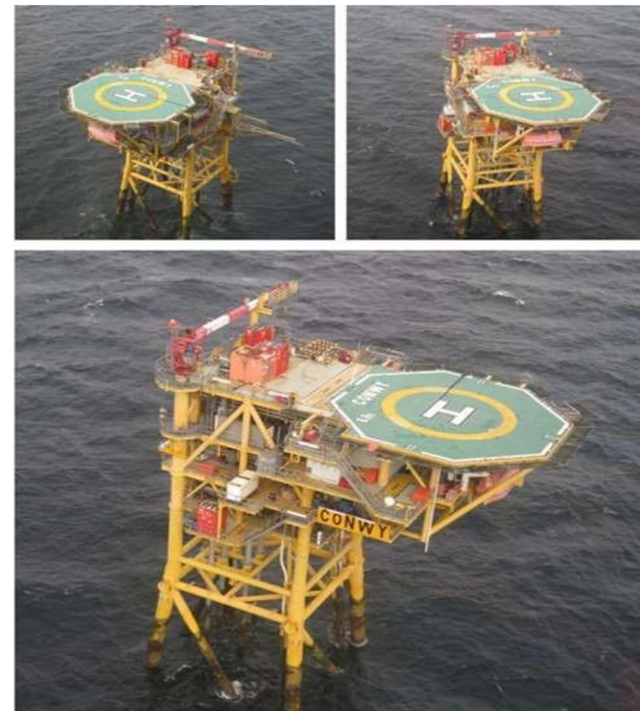
5:1 NE, SW & NW access platforms
