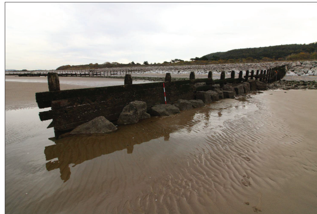
Plate 5: Timber groyne with stone foundations, looking southeast, scale 1m.
