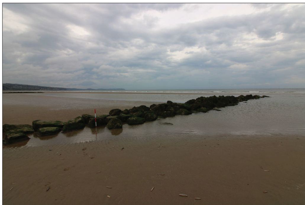
Plate 4: Stone groyne foundations looking northwest, scale 1m.
