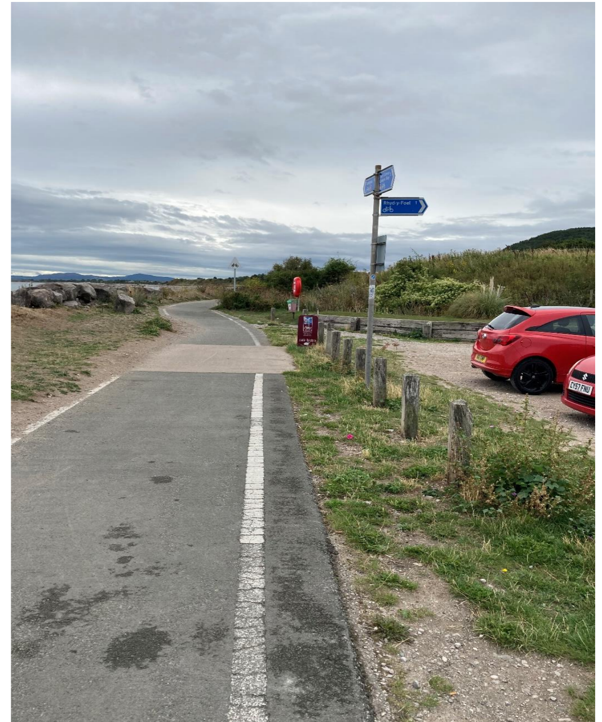
Figure 20.8: Photograph of the combined Coastal Path and National Cycle Route 5 within the land use and recreation study area.
