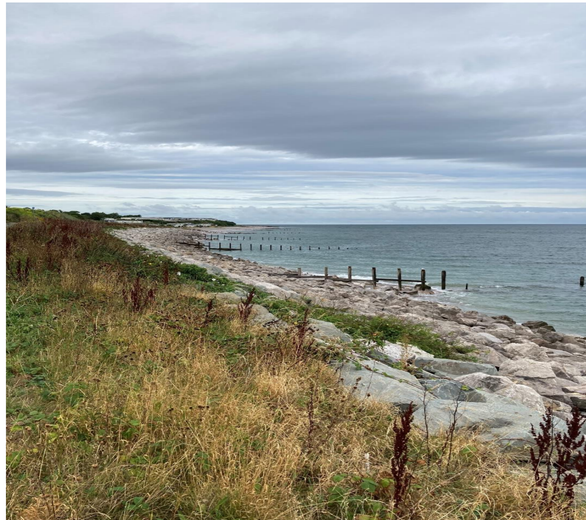
Figure 20.7: Photograph of the coastal defences located within the land use and recreation study area.
