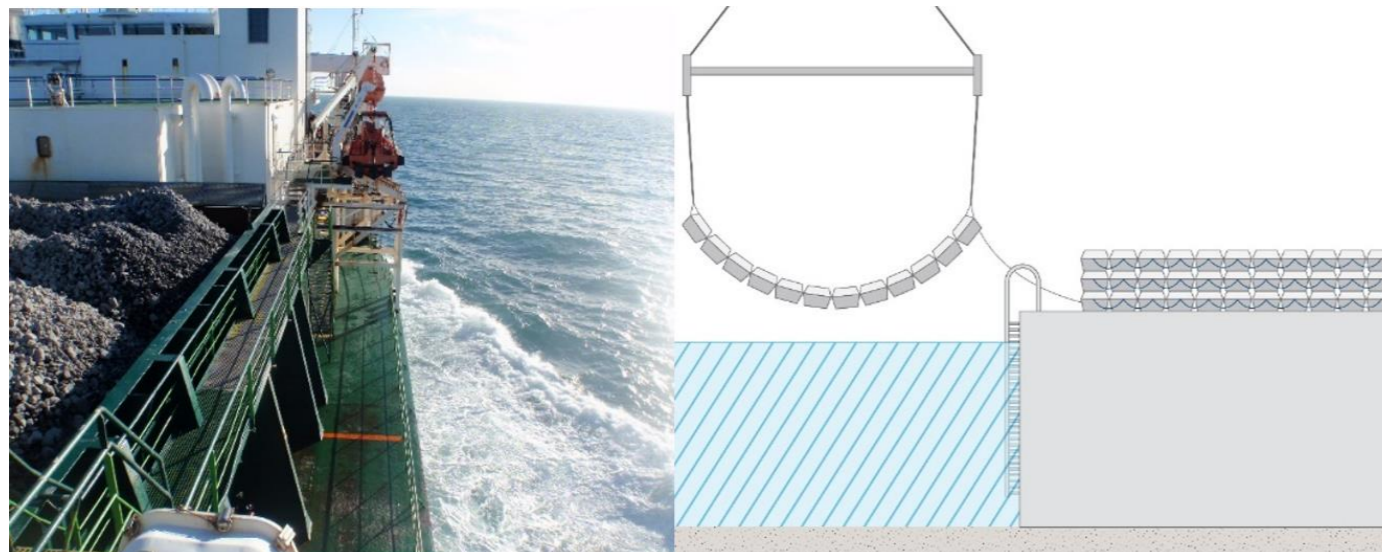
Figure 3.11: Illustrative scour protection types (Left: delivery of rock to EnBW’s Hohe See offshore wind farm; Right: concrete mattresses).
