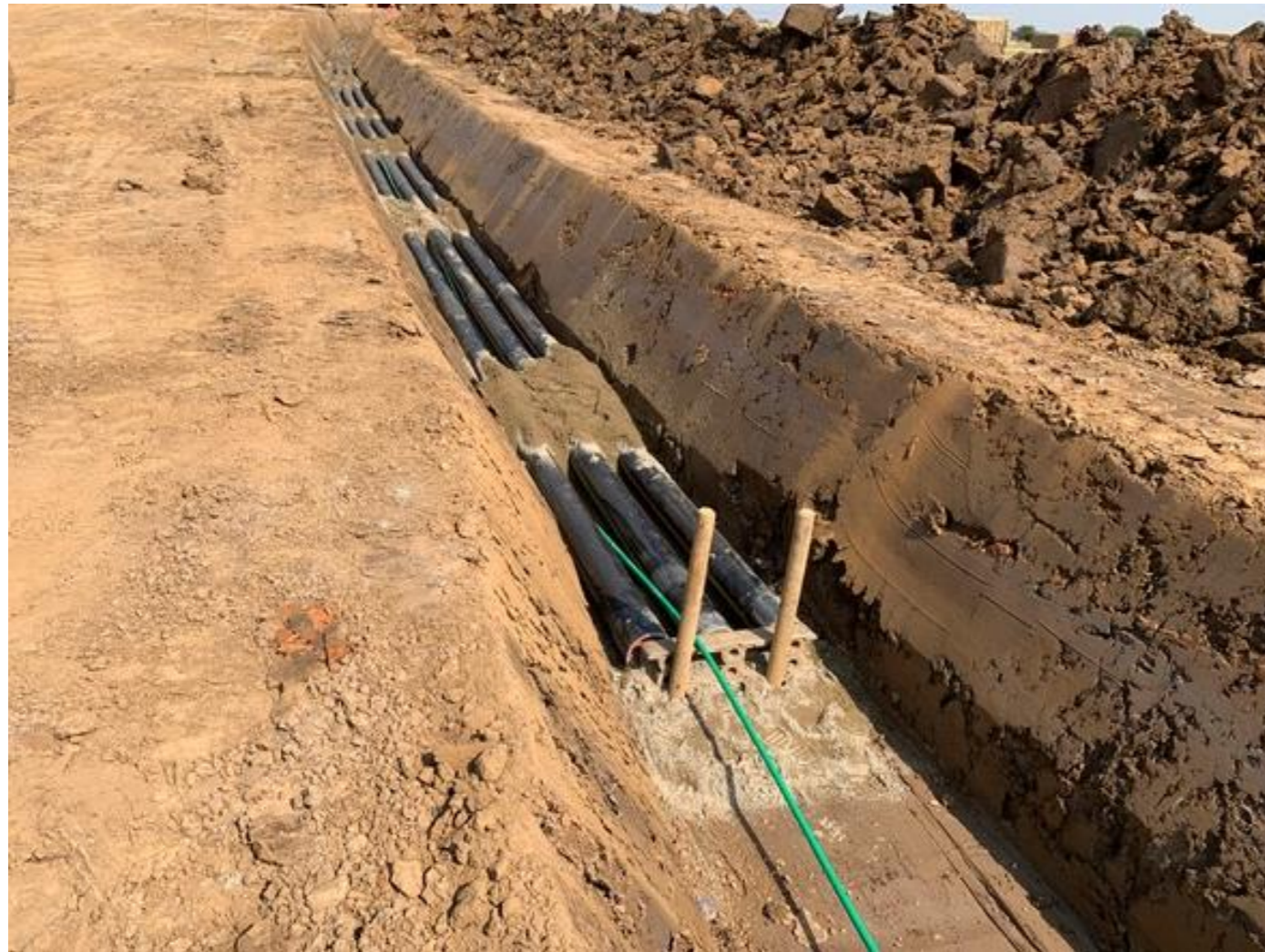
Figure 3.18: Example of an onshore export cable trench.
