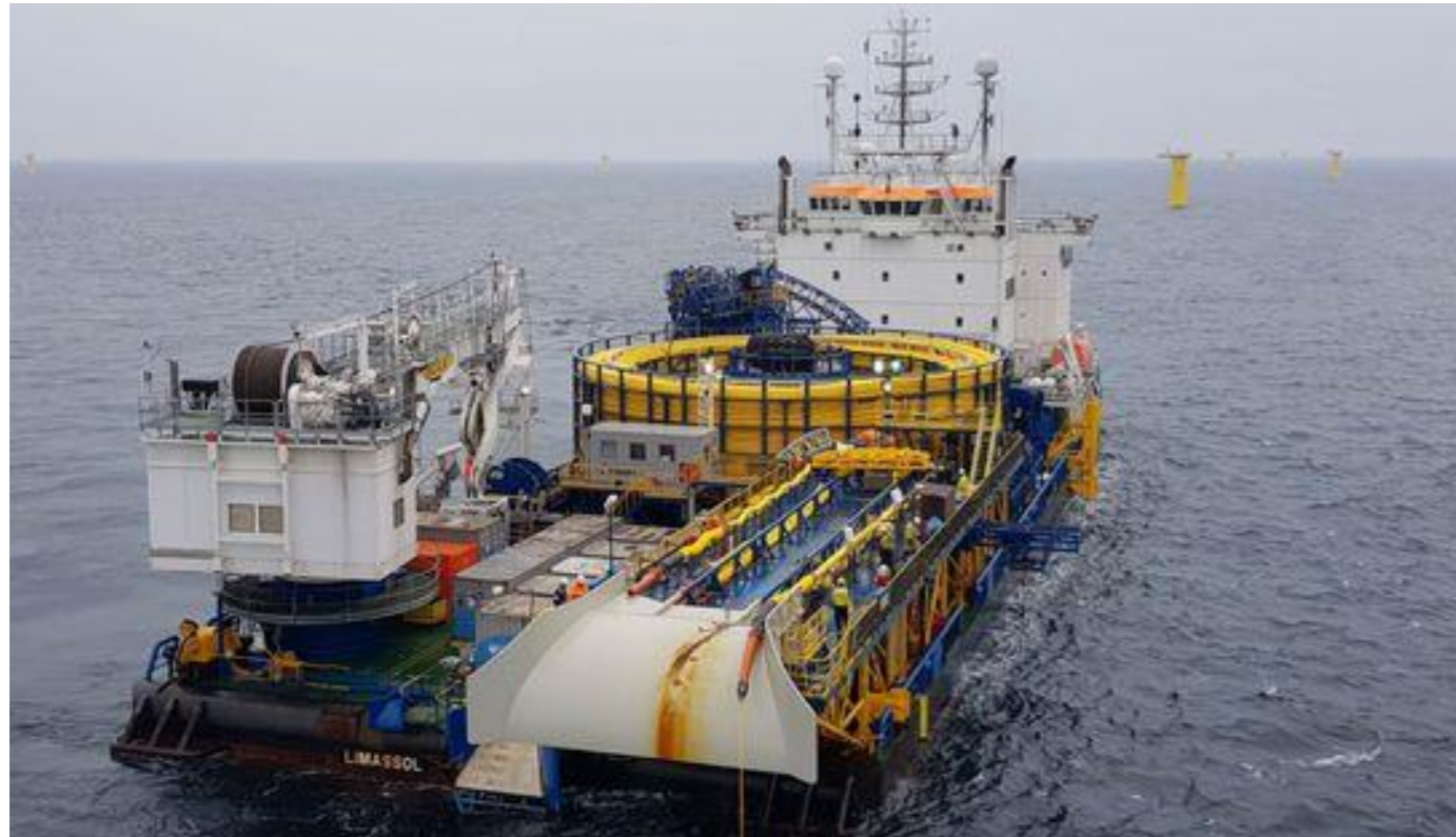
Figure 3.12: Example of inter-array cable installation at the EnBW Hohe See Offshore Wind Farm construction site in the German North Sea.
